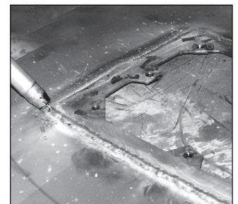
\* If using the frame on the outside of the duct, a continuous liquid tight weld is required. Care should be taken to not warp the frame when welding.
