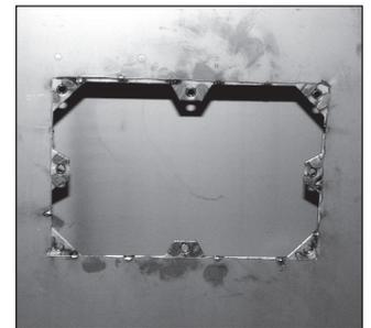
6. Correctly installed frame.
